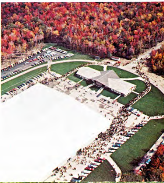
The Tabernacle and Administration Building Complex.
